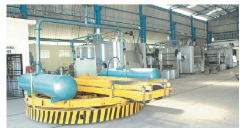
In-House Heat Treatment
